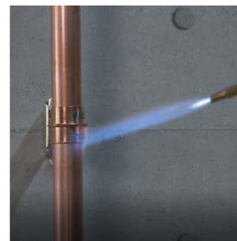
To fix the pipe support completely, brazing is necessary.
