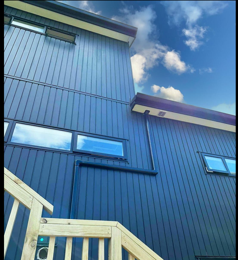
Installed by Harrison Air Conditioning
